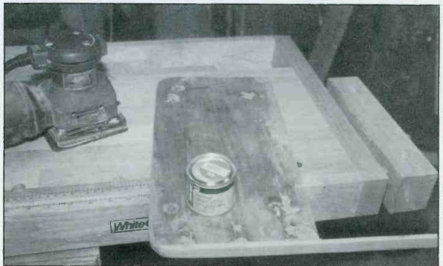
Maple strips replaced the damaged sections that were previously removed. Soft punky areas of the pine baseboard have been dug out with a sharp penknife, filled with wood filler, and sanded smooth.
